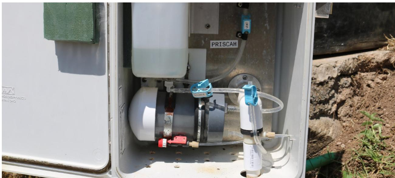
A close-up of an automated chlorine dosing device installed at a water system. Such systems help ensure consistent water disinfection, improving the safety and reliability of community water supplies.
